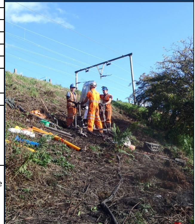
Above & Below: Modular Window Sampling Rig
